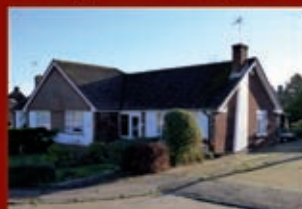
CUCKFIELD 2 bed semi-detached bungalow £350,000
