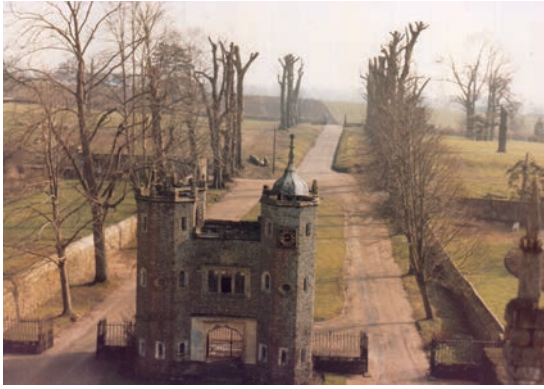
View from the roof of Cuckfield Park when the damage had been cleared
